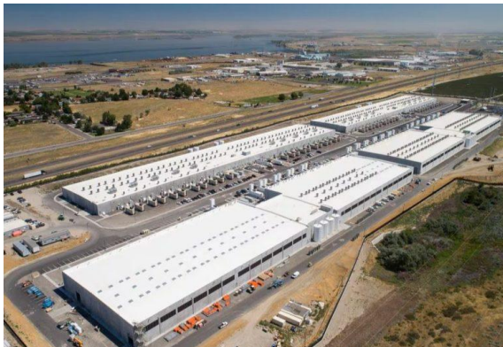
Figure 15: Amazon Web Services (AWS) Data Centre in Boardman, Oregon
