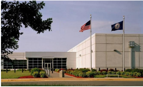
Figure 16: Linton Hall Facility
